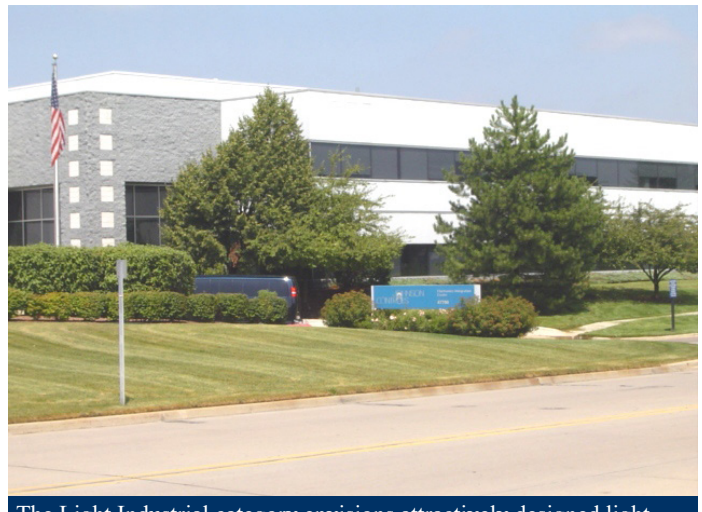
The Light Industrial category envisions attractively designed light-manufacturing, technology, research and office uses that provide jobs and boost the local economy.
